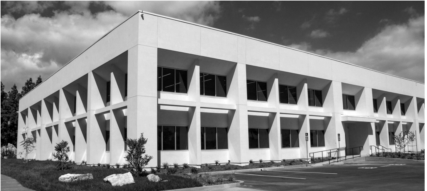
City-owned building located at 12616 183rd Street
