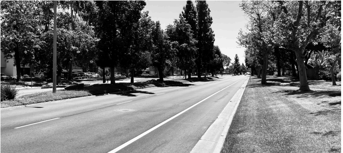
Bloomfield Avenue Street Improvements
